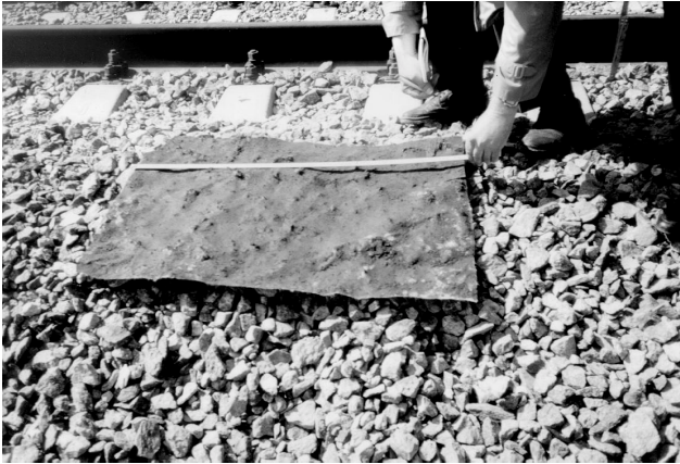
Figure 4. Excavated sample of geotextile with some old ballast
