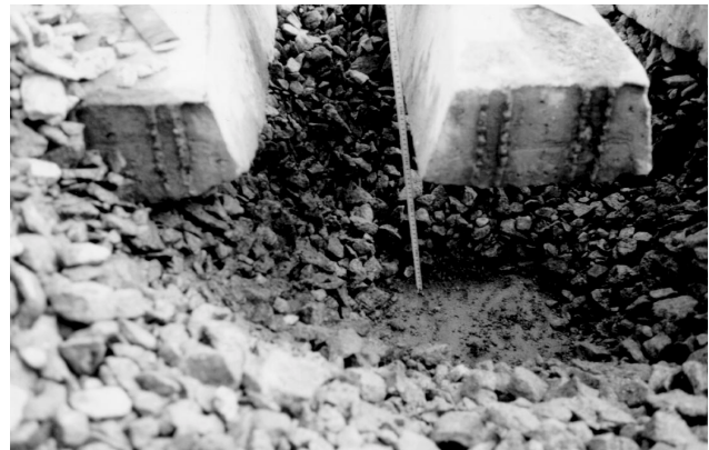
Figure 3. Excavation from under the track
