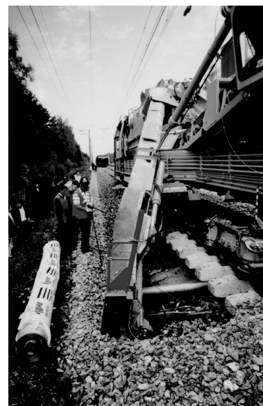
Figure 2. Track renewal with specialised equipment
