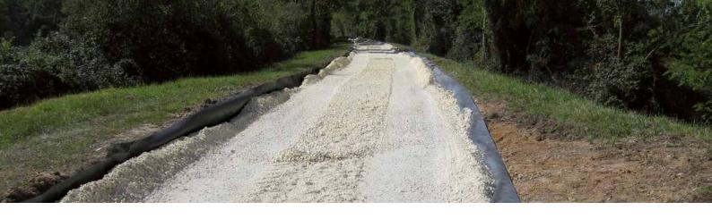
The new Plantex® RootProtector is a strong, water-permeable root barrier suited to both vertical and horizontal applications. It is manufactured from continuous PP filaments that are spun and laid down as a web which is thermally and mechanically bonded at filament crossover points.
