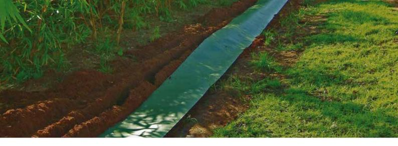
DuPont™ Plantex® RootBarrier is the ideal solution to control plants with aggressive root systems such as bamboos and pyracantha. It is particularly recommended for critical applications such as protecting buried linear networks: cables, water piping, pavements, paved areas, roads, water and sewage networks.
