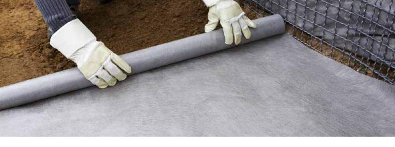
DuPont" Plantex® Geoproma® is a 100 % thermally-bonded polypropylene, rot-proof geotextile. It avoids the loss of bedding into the subsoil, and prevents soil from migrating into the drainage system. Plantex® Geoproma® ensures your construction stays even- for a long time. Its filtration characteristics ensure continuous drainage. It is chemically inert, does not deteriorate and is environmentally friendly.
