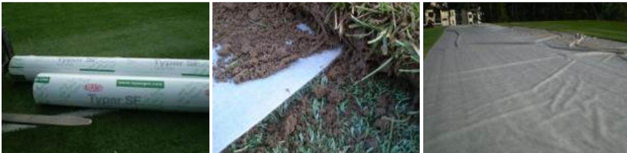
From left to right: rolls of DuPont™ Typar® ready to be installed; detail of the ground with DuPont™ Typar® geosynthetic applied; application of DuPont™ Typar® geosynthetic on the football field; photos by Bruno Marabotto, all rights reserved.
