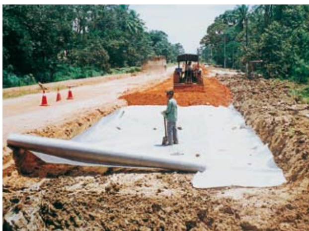
Road construction, Malaysia
