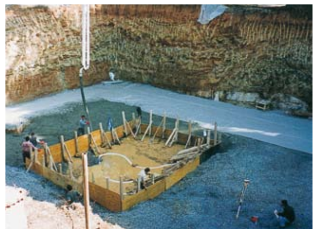
Building construction, Turkey
