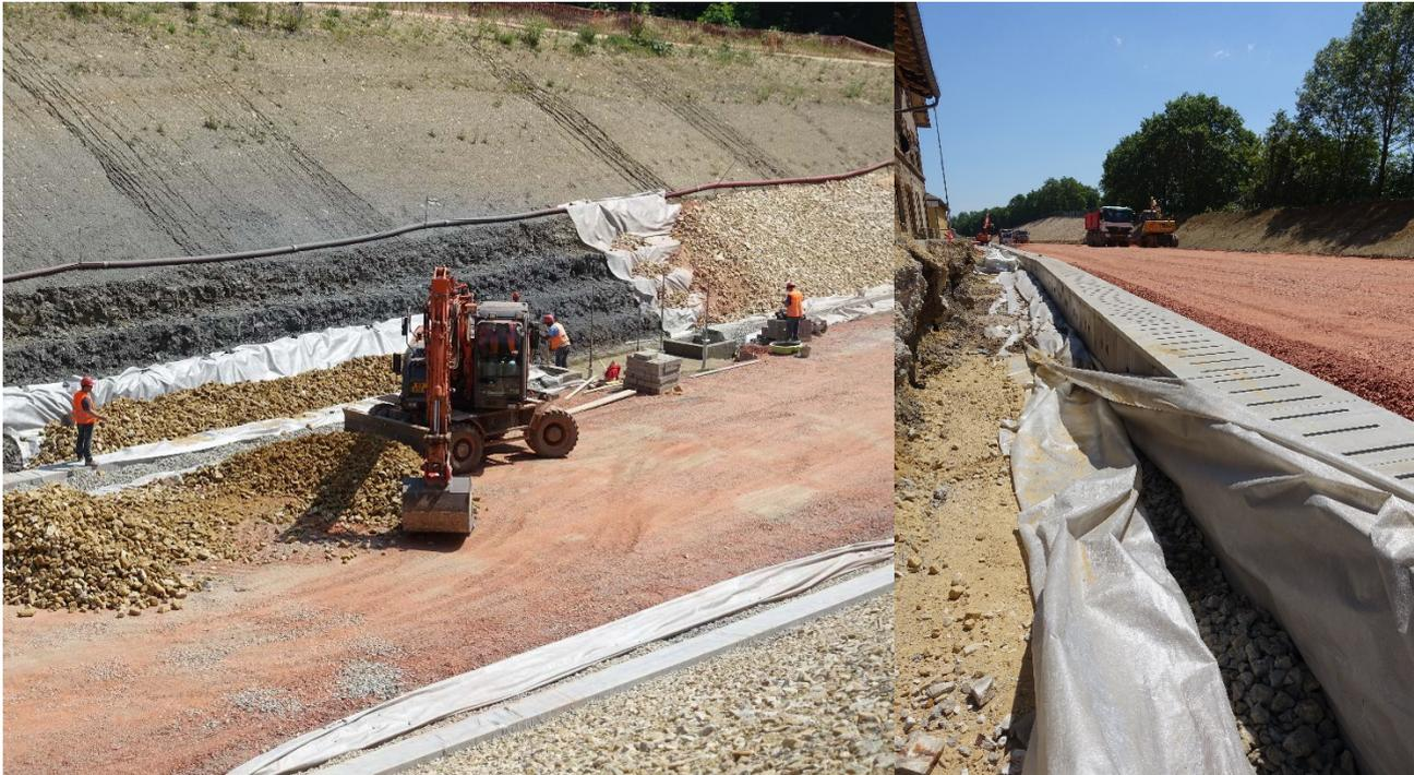
**Project :** Doubling of the railway line between Luxembourg and Sandweiler-Contern. The preferred choice of geotextile was Typar® SF for separation, stabilization and drainage.
